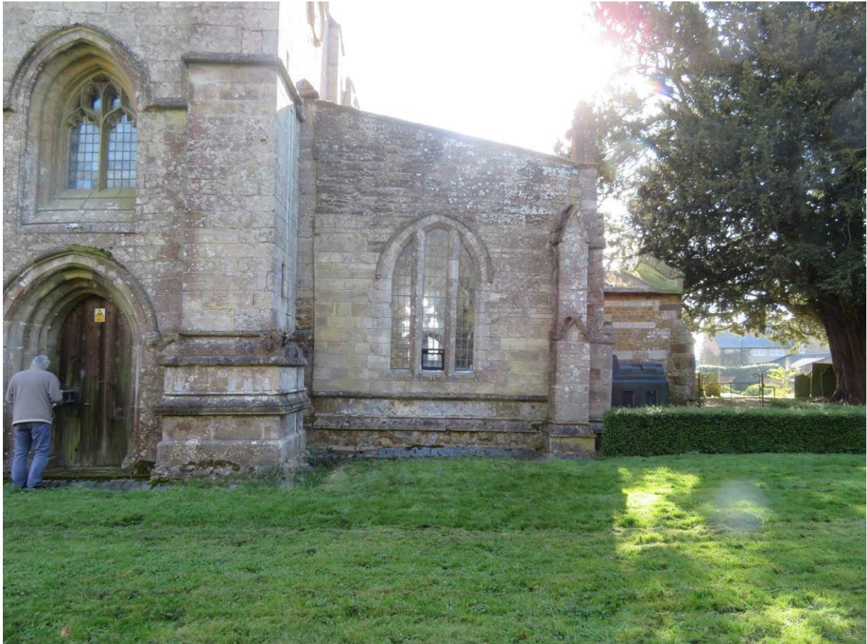
Photograph 16: Settlement of the west wall of the south aisle is obvious
