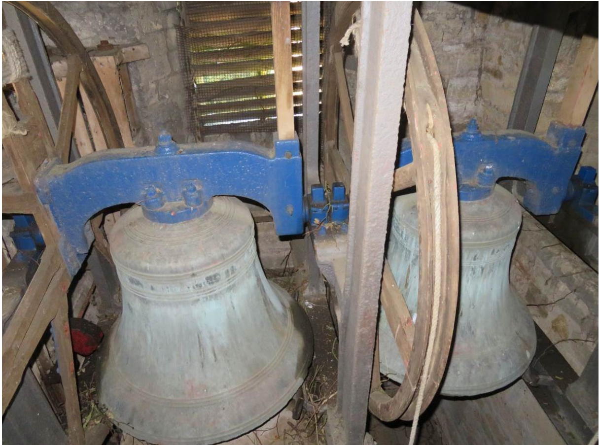
Photograph 20: Part view of bell frame with two larger bells swinging north south
