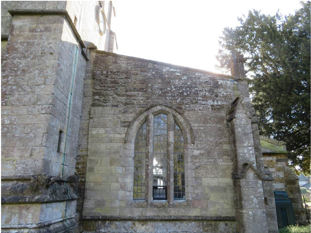
Photograph 17: Re-build to head of gable and which is relatively horizontal
