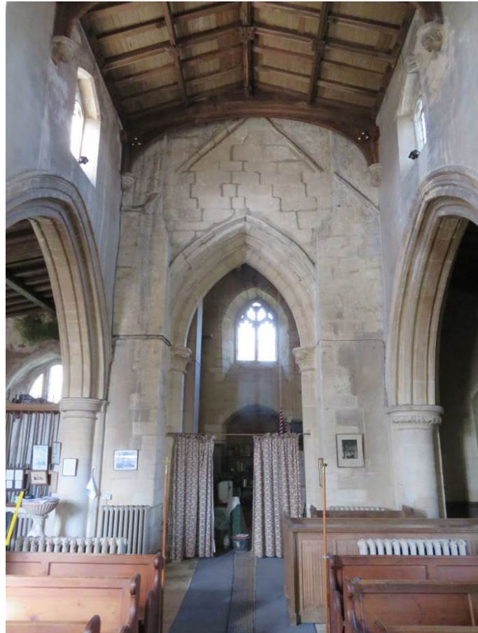
Photograph 28: Internal face of east face of tower with cement pointed cracks
