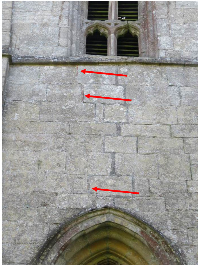
Photograph 19: Crack to west elevation of tower with tiles slips used (highlighted)
