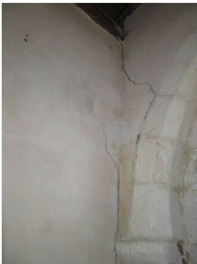
Photograph 12: Crack to east side of door arch to porch
