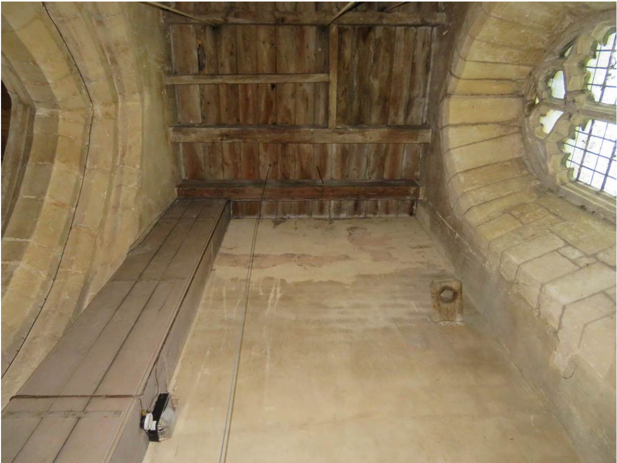
Photograph 25: Plastered walls to lower stage of tower with failure to high level south wall
