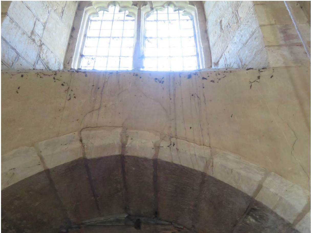
Photograph 27: Minor cracks over west door arch
