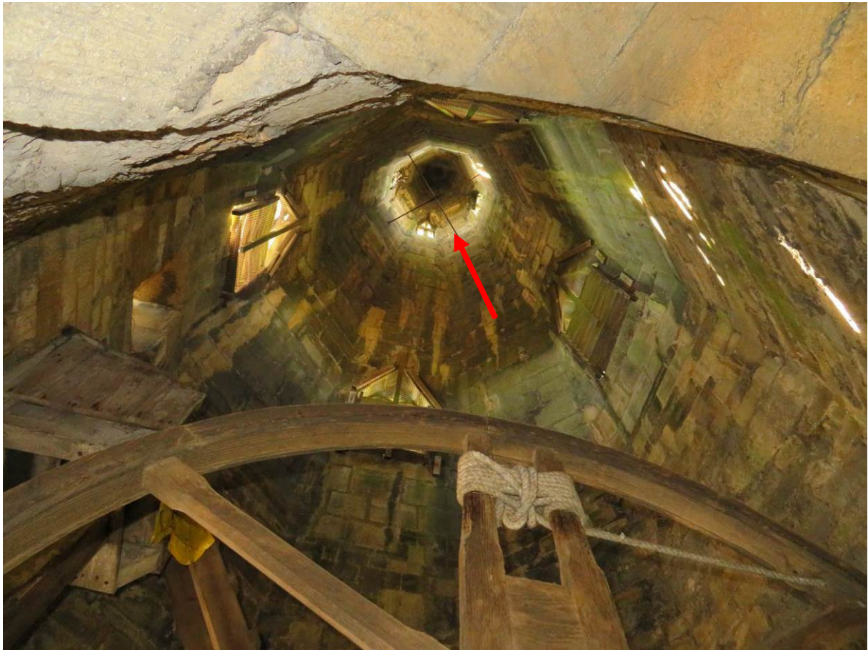
Photograph 23: View up spire with cross tree apparent and highlighted
