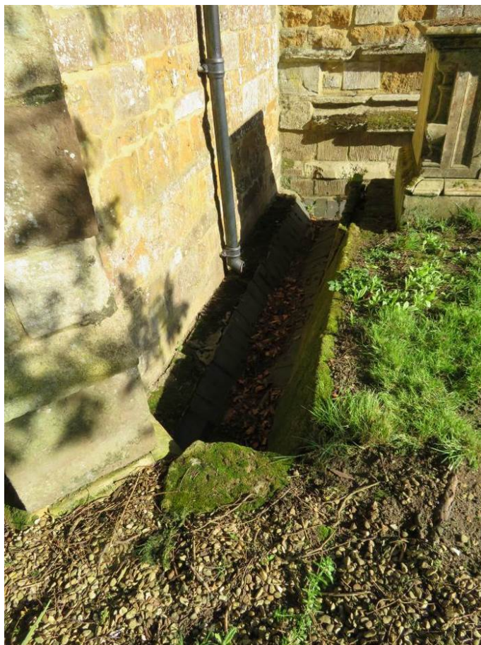
Photograph 13: Drainage collection channel to east side of porch
