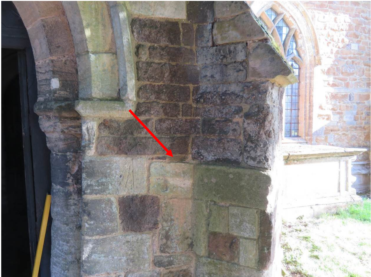
Photograph 15: Ironstone re-building over limestone to porch with levelling course highlighted
