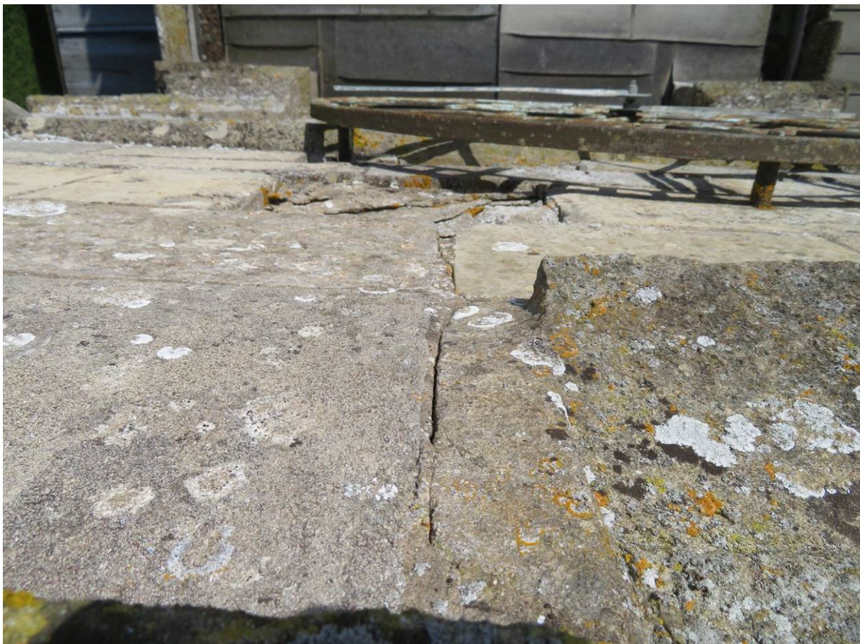
Photograph 22: Open joints parapet as seen from the tower gutters
