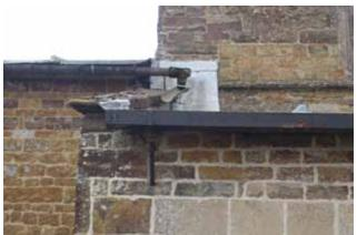
RWP-6 North clerestorey, east end. 1791 lead hopper [blocked] with poorly fixed corroded cast iron rwp discharging over aisle roof.
