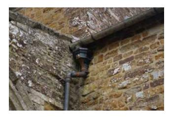
RWP-3 Lead hopper with corroded cast iron downpipe to open and blocked surface water gulley. This is the cause of significant damage to the external and internal fabric.
