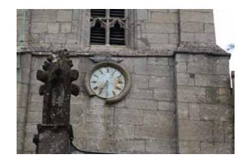
Offset stringcourse with open joints. The line of the stringcouse was amended when the Chapel in the South Aisle was built. These is a significant issue at the junction of the South Ailse parapet gutters abutment to the tower which is causing the internal green mould and this requires urgent attention.
