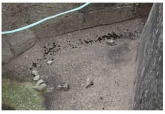
There are areas of erroded stone and poor plastic repairs which are failing.
