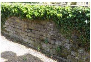
North: Retaining wall partially collapsed at west end.
