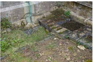
RWP-I Lead hopper to Aisle with cast iron downpipe. Lead hopper to Porch dated IM 1795. Very corroded cast iron rwp to water but with an in adequate temporary outlet. This is the cause of significant damage to the internal fabric.
