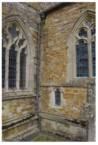
RWP-4 Small lead hopper dated 1795. Lead downpipe with taped up repairs. The pipe is in poor condition and very distorted. Discharges to an open channel in poor condition with a blocked gulley. Significant damage being caused to the base of the adjacent buttress.
