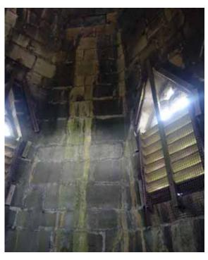
Significant efflorescence at the base of the spire [under the line of the tower gutter] .
