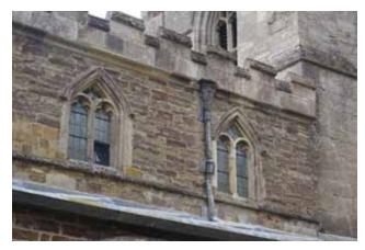
RWP-8 South clerestorey, west end. 1791 lead hopper with lead rwp discharging over aisle roof.
