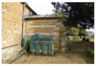
RWP-2 Cast iron downpipe to open and blocked surface water gulley. This is the cause of significant damage to the internal fabric.
