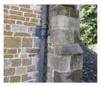
RWP-5 Short corroded cast iron down pipe and gutter section discharging to Aisle roof.
